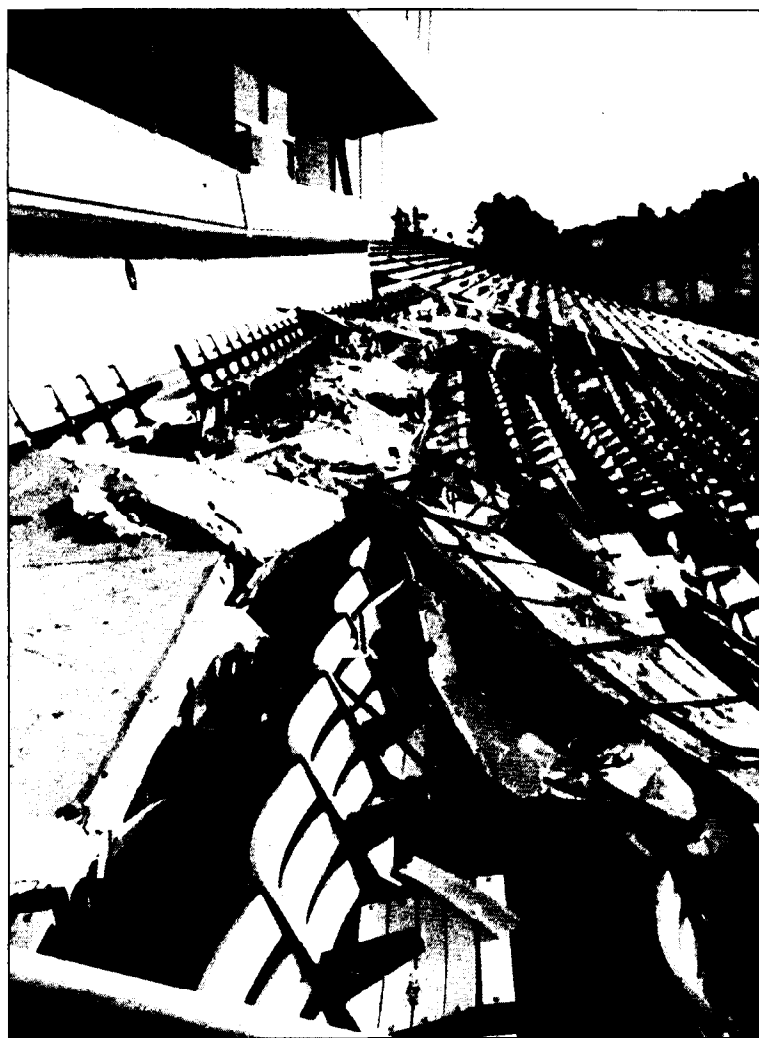
Nicholls State University in Thibodaux, Louisiana, suffered more than $500,000 worth of damage from Hurricane Andrew, including $126,000 to John L. Guidry Stadium. The concrete facade between the third floor and the roof of the press box was ripped off by the storm, and falling debris destroyed 52 chairback seats.
